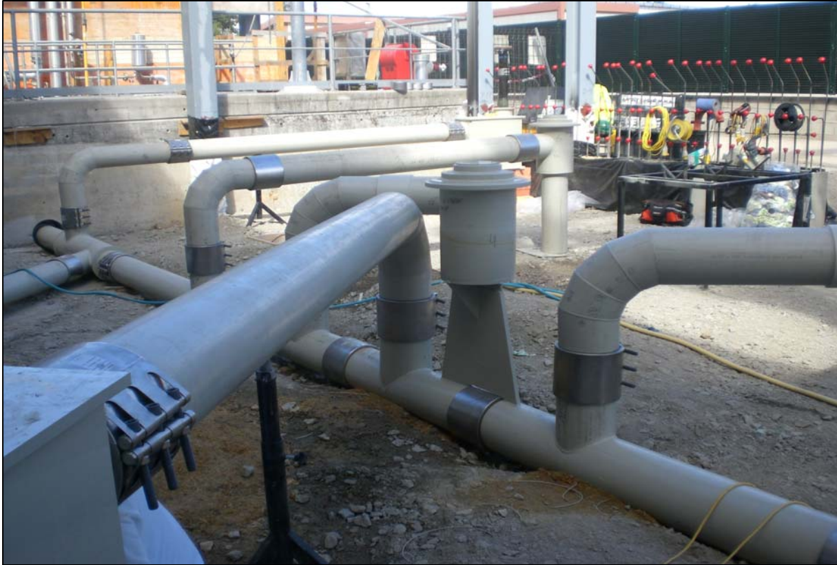
(Dual Contained Pipe, GRE Internal Pipe With Polypropylene Outer Pipe)
