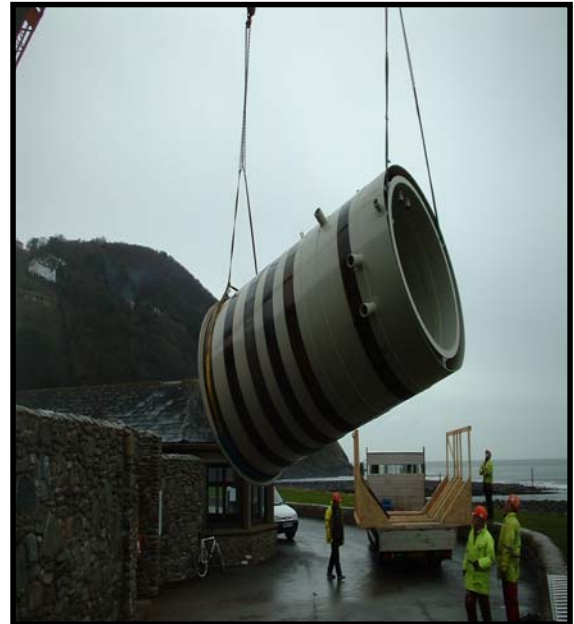
Pictured: Above: PipeX chamber being offloaded and lowered into position.
