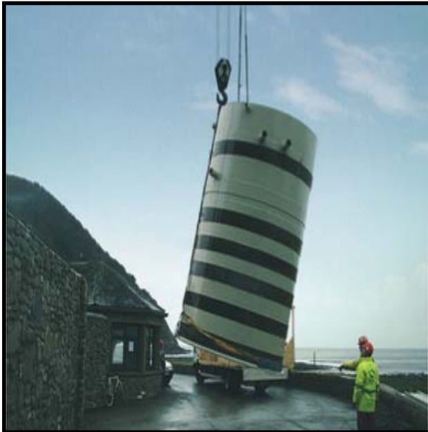
Pictured: Above: PipeX chamber being offloaded and lowered into position.
