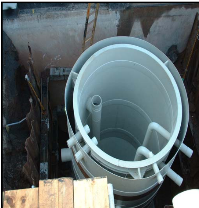
Pictured: Above: PipeX chamber being offloaded and lowered into position.
